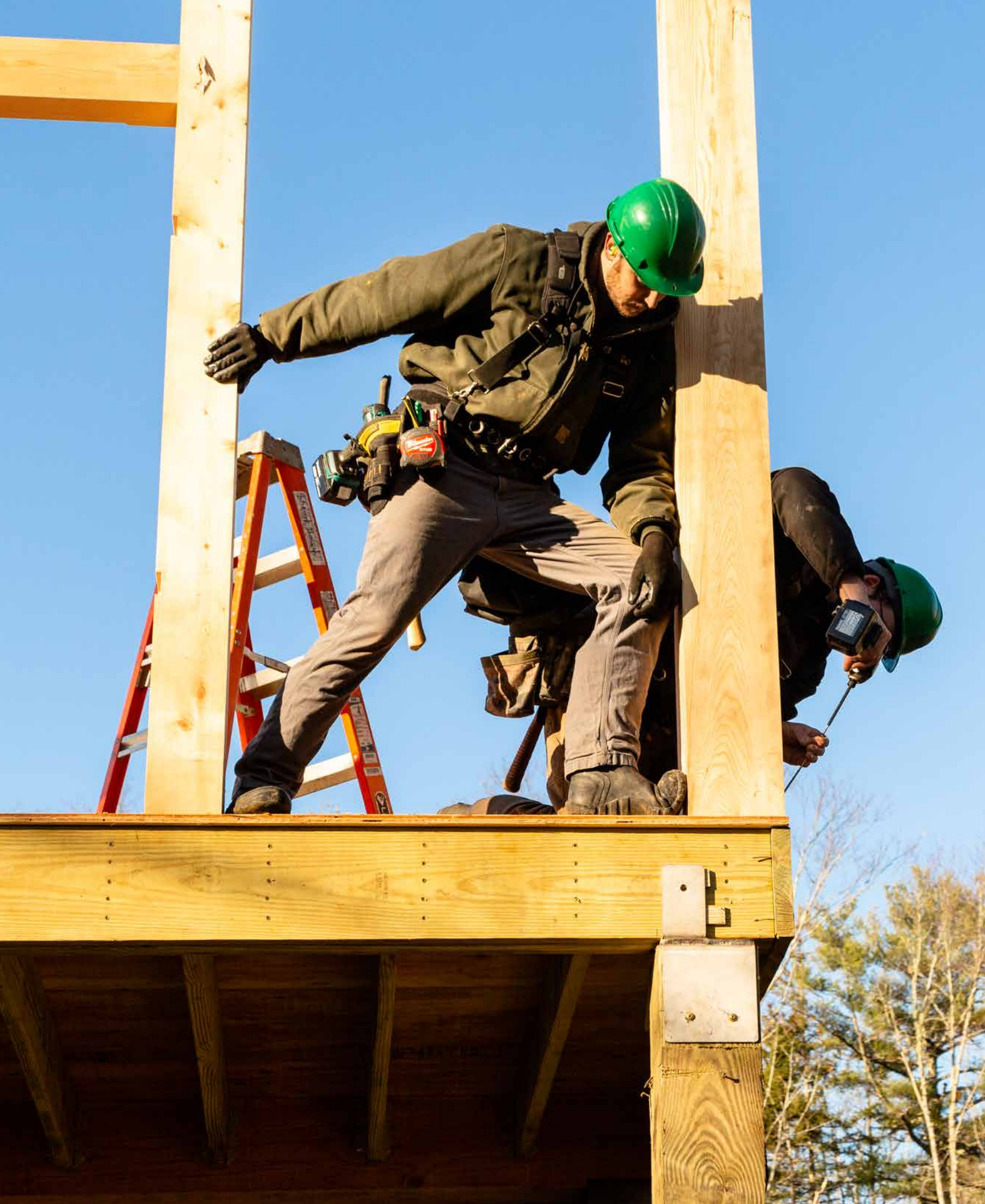
Left: The assembly team from Shelter Institute anchors hand-hewn hackmatack beams to the cabin platform. Above: Nancy Kennedy, vice president for Camp Chewonki, and Emily Bell-Hoerth, director of Camp Chewonki for Girls, visit the first full-sided cabin on a frosty January morning. Below: The post-and-beam design requires meticulous planning, cutting, and assembly.
